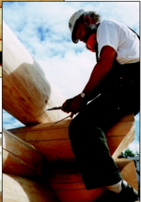
Hold the scribe gently with both hands, keeping the level bubbles between the lines.
