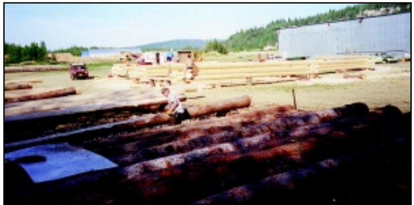
Prebuilding the log walls at a convenient place before reassembling at the final homesite. The logs are peeled just before use to keep them in good shape.
