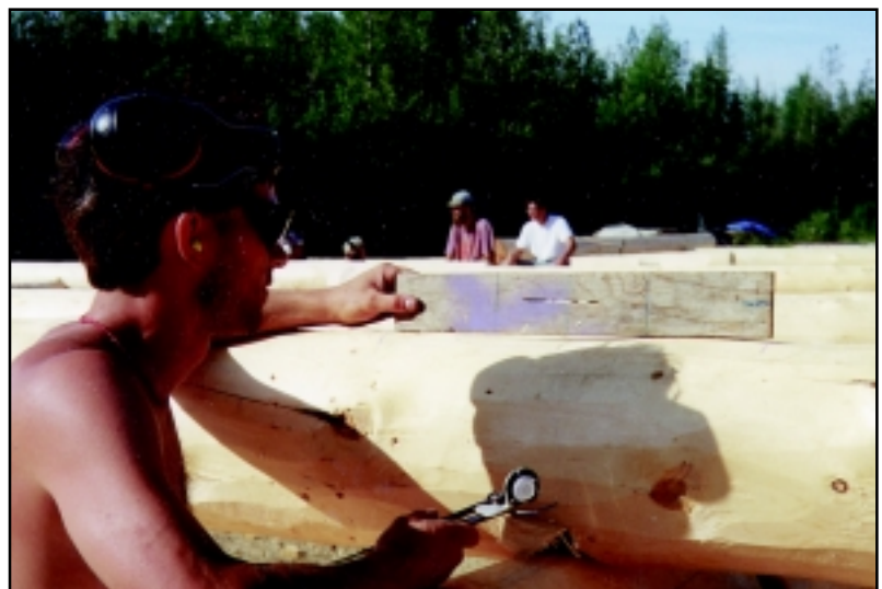
Using a layout board to mark the log for a scarf. See drawing #3, page 37.
