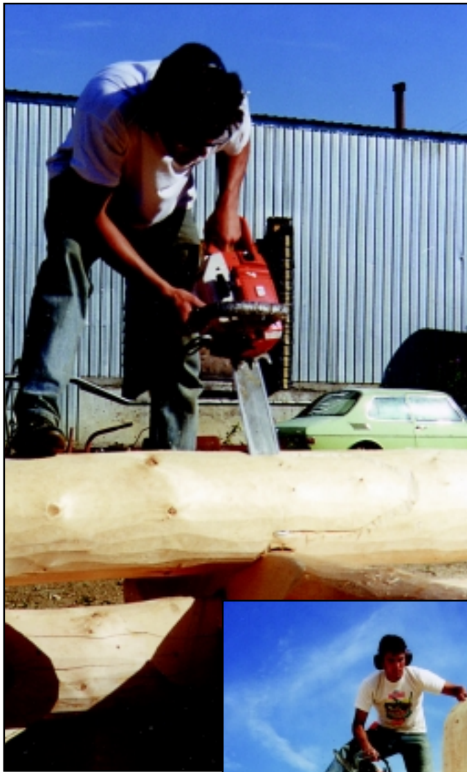
cutting the scarf
