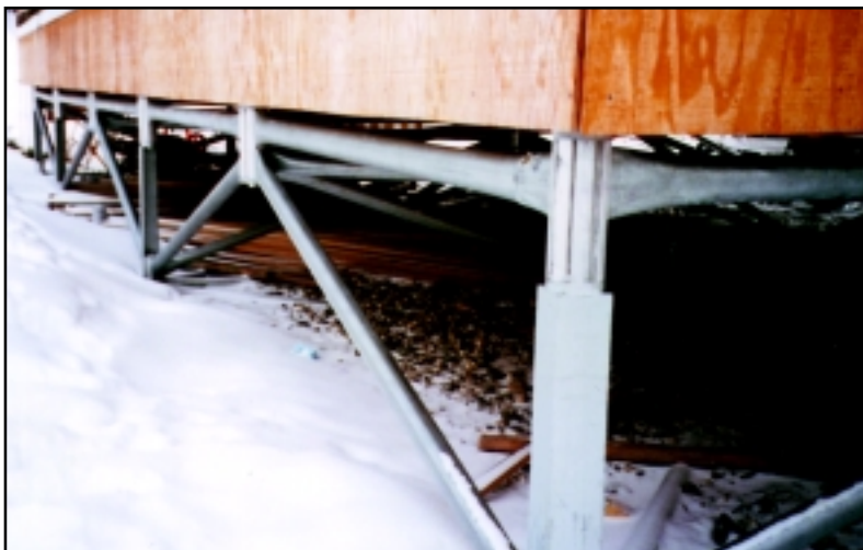
The Triodetic brand space frame is one option for building on permafrost.
